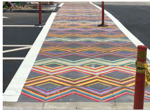
Crosswalks-Ennis Flint Traffic Patterns Thermoplastic Inlay with pattern lasts up to 10 years with normal wear
