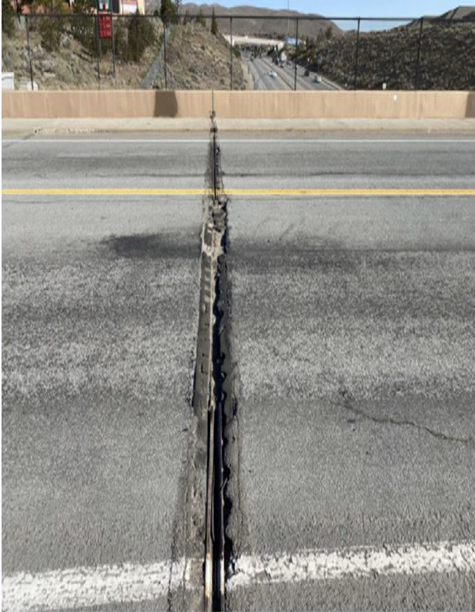
(Figure 1. Failure of Summit Ridge Drive Bridge West Expansion Joints
