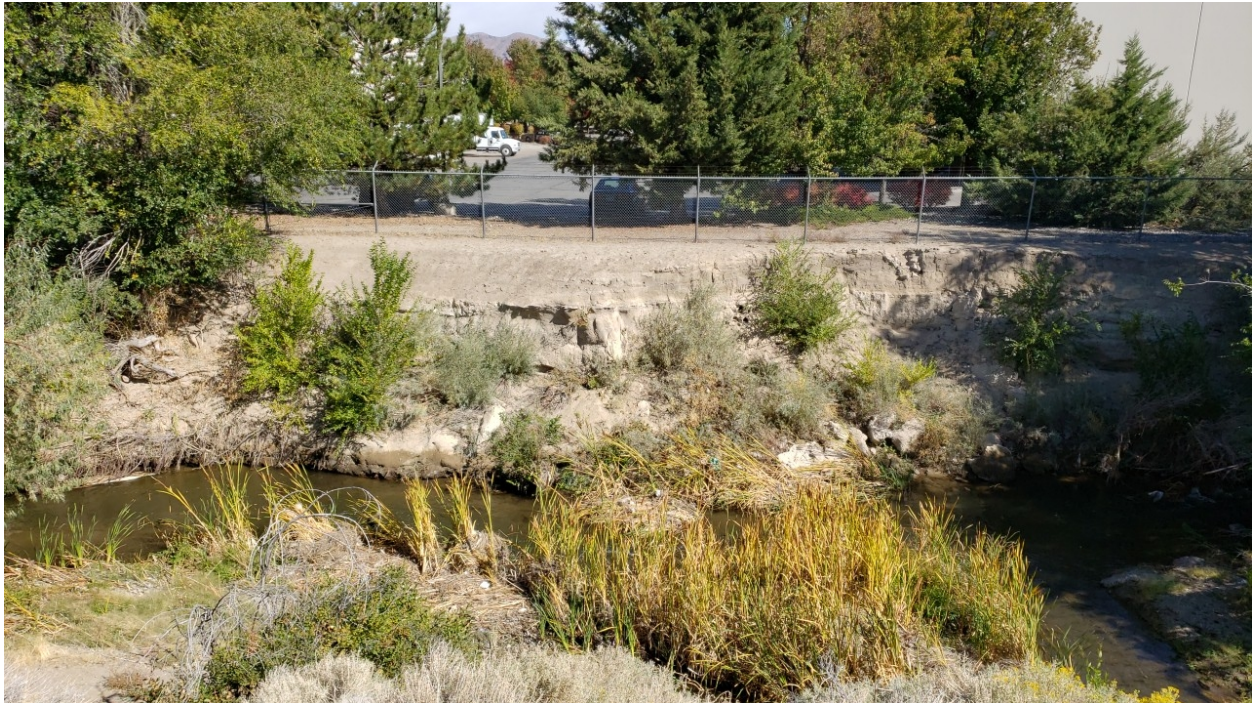
Figure 1: Bank erosion along the airport's east perimeter fence
