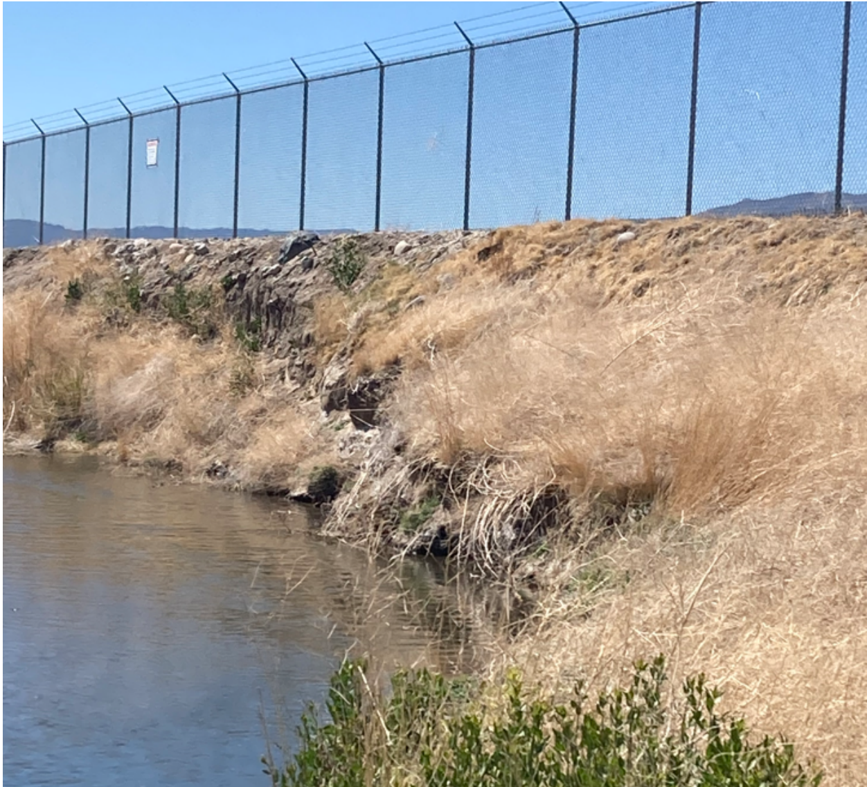
Figure 2. Erosion encroaching toward airport security fencing
