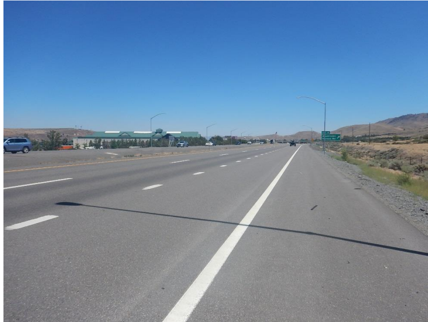
VIEW OF INTERSTATE-80 FACING EASTERLY
