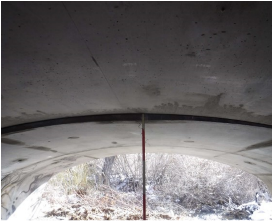
Figure 3. Sag evident in Arch Segment No. 8
