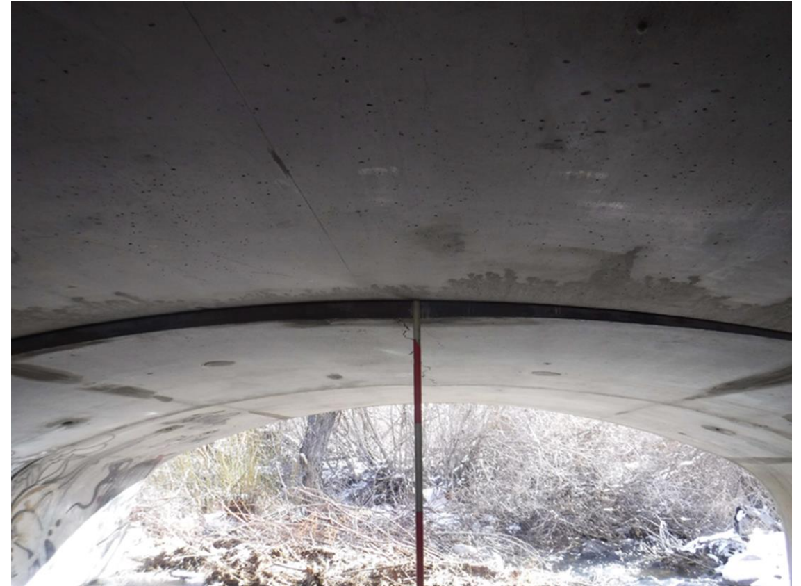
Sag in the top of Arch Segment No. 8
