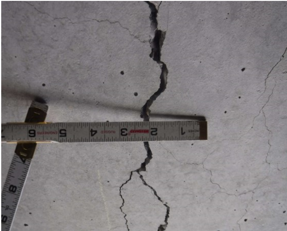
Figure 4. Flexure cracking in crown of Arch Segment No. 8
