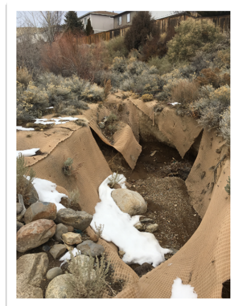
Figure 2. Channel erosion
