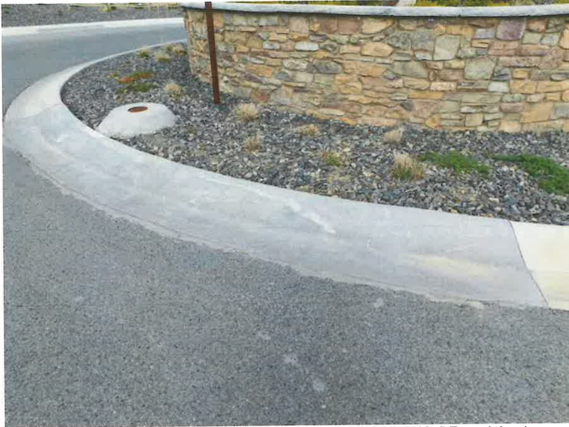
Figure 20 – New Concrete Curb observed around "The Cliffs" Roundabout
