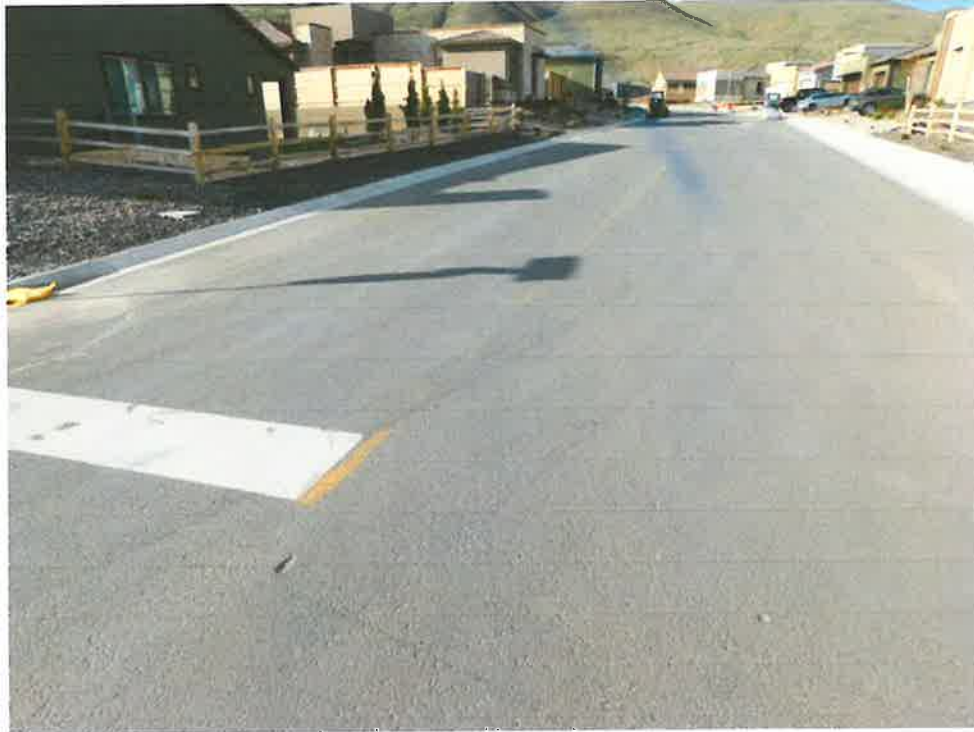
Figure 28 – Fading Yellow Roadway stripe and stop bar which should be re-striped.
