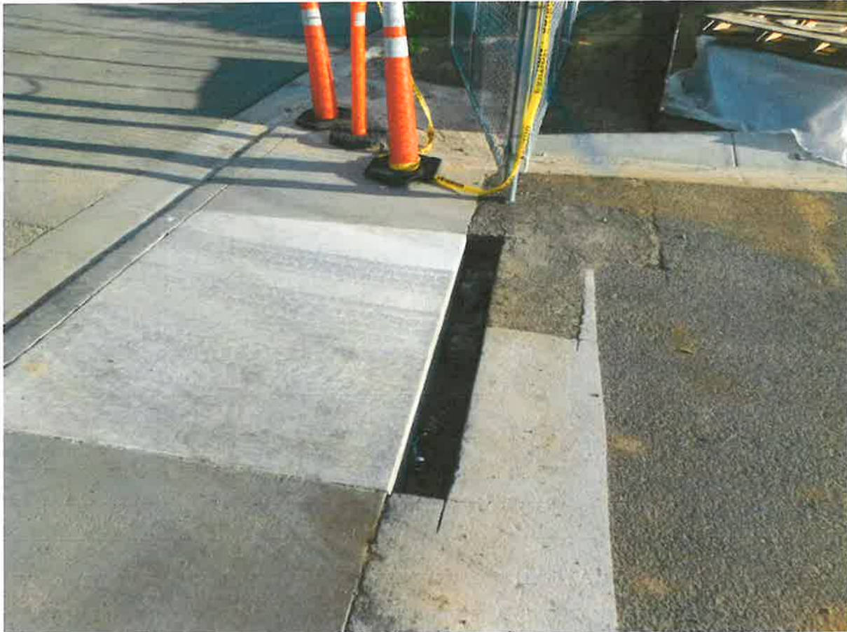
Figure 32 – Open sawcut area at start of Blue Pinion Drive during May 2023 site visit was severe hazard. This has since been filled in.
