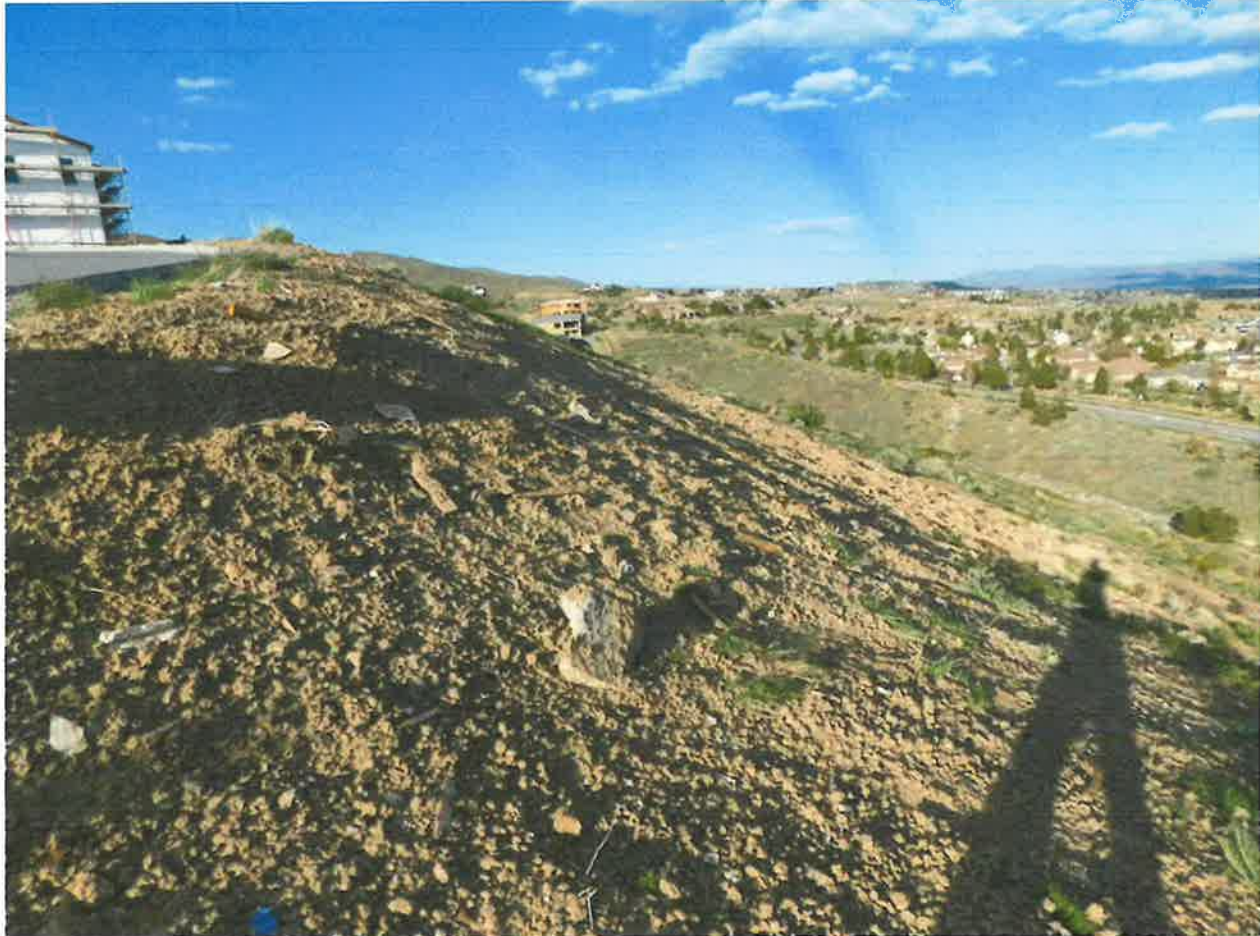
Figure 31 – Another view of the Hillside Erosion Issue. Installation of Sediment Rolls and Re-Seeding would be the recommended fix; however, given the previous re-seeding issues, installation of rip rap at this location may be the preferred fix. There is a lot of trash and debris at this location that should be cleared as well.
