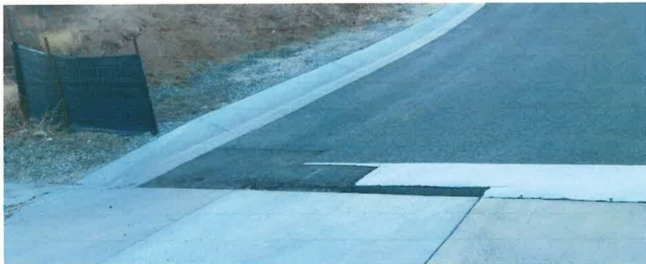
Figure 33 – Open sawcut area at start of Blue Pinion Drive during May 2023 site visit was partially filled in During January 25, 2024 Site Visit. Note that hole was filled with Cold Patch which is already showing signs of failure. This is a temporary or "Band-Aid" Fix, which by my understanding was not performed by Toll Brothers. A long term fix for this section would be to remove section and replace asphalt section with hot mix asphalt at the very end of construction activities, or sawcut entire section and re-pour with concrete. Due to mobilization costs it would be prudent to fix this spot in the future when other hot mix asphalt paving is occurring in the area.
