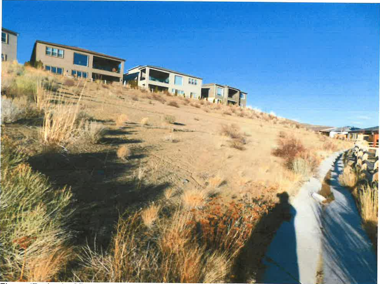
Figure 47 – Lack of Reseeding, Lack of Slope Stabilization Treatments, Erosion Issues, and Trash and Debris in Gutter still prevalent in open space between Graycliff Lane and Wild Skies Way. Photo Taken January 25, 2024.
