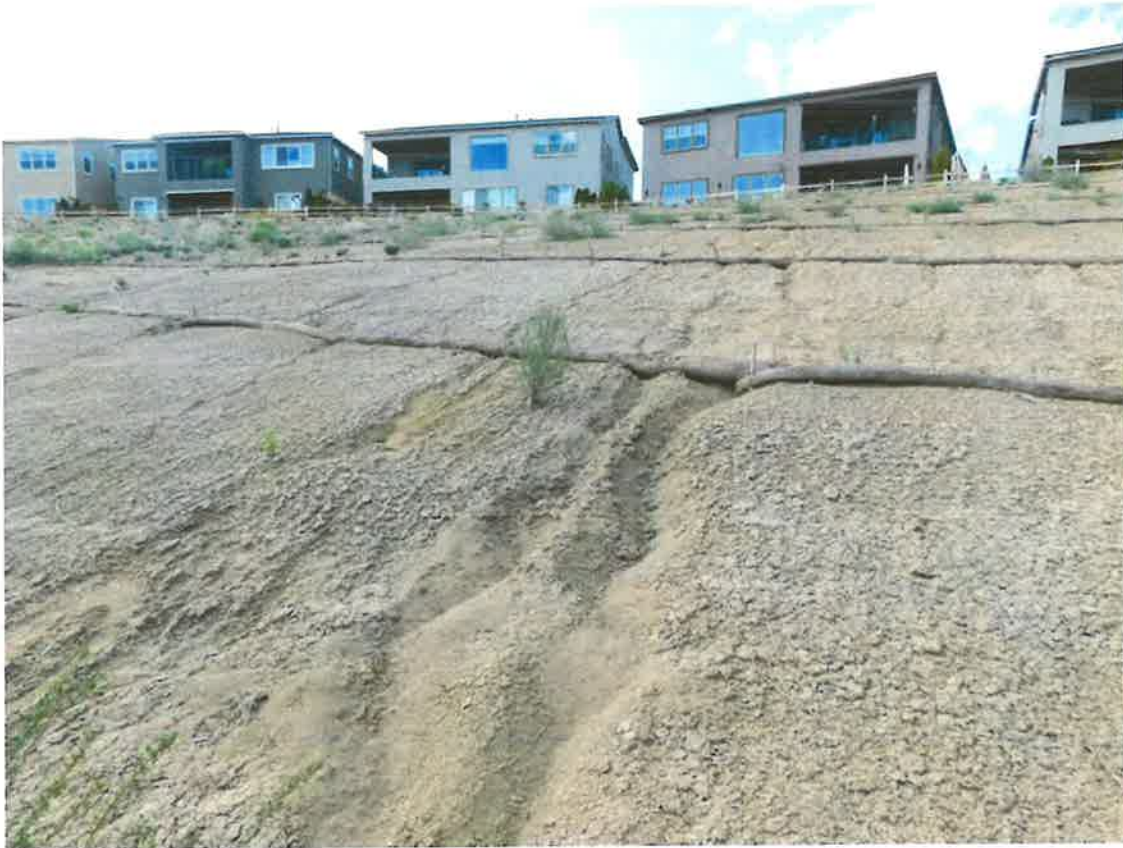
Figure 9 – Lack of proper Re-Seeding / Revegetation has caused erosion issues. Photo taken of Open Space Area which runs between the corner of Wild Skies Way / Graycliff Ln and "The Cliffs" Roundabout.
