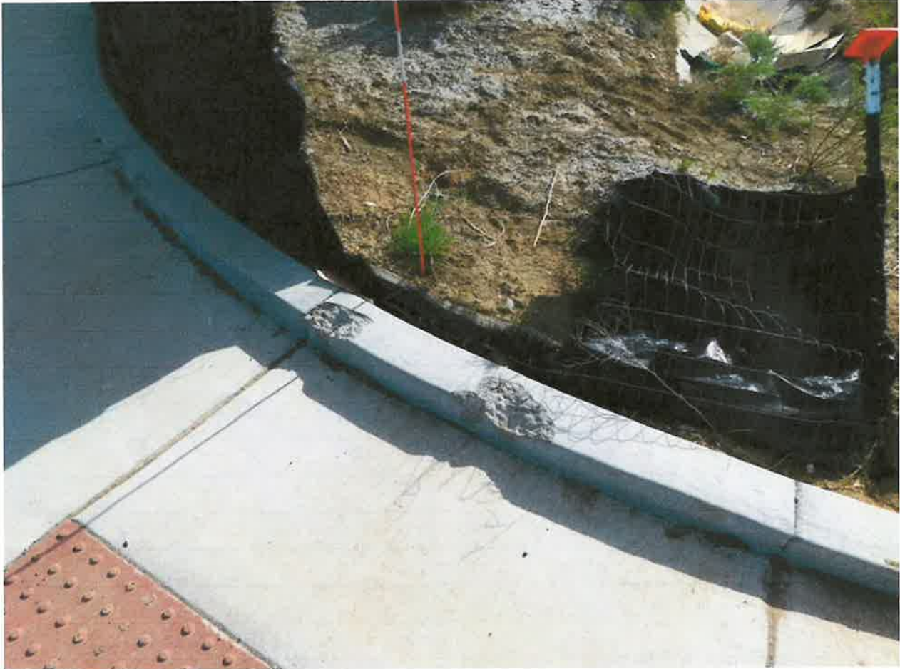
Figure 41 – Damaged Curb at Corner of Wild Skies Way and Graycliff Ln Recommend Replacement of this section. Silt fence has been damaged and should be replaced during construction as well. Note that the silt fence has been removed as of January 2024; however, the
