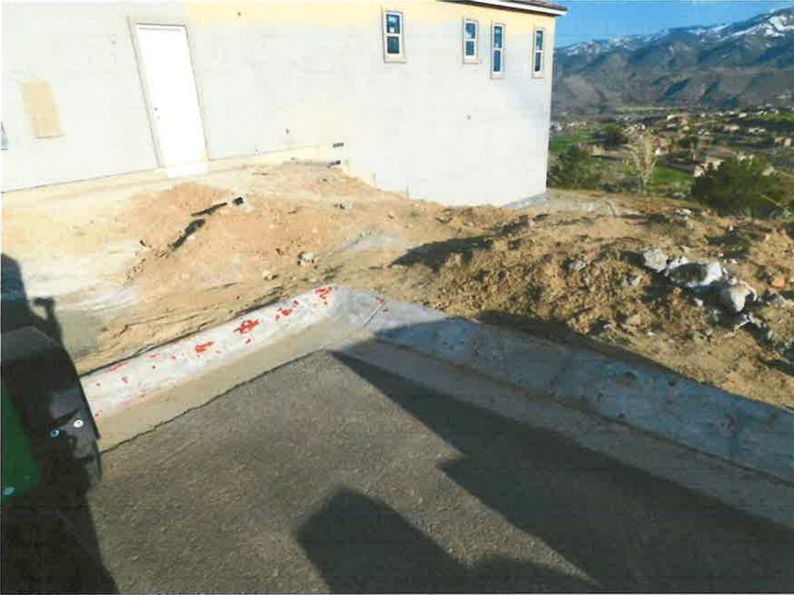
Figure 39 – Red Striping at Fire Turnaround at the end of Blue Pinion Dr is almost non-existent and needs to be restriped.
