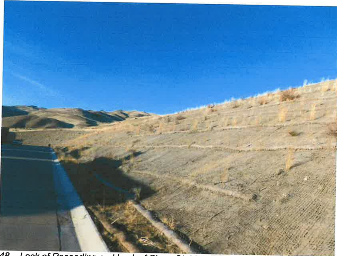
Figure 48 – Lack of Reseeding and Lack of Slope Stabilization Treatments still prevalent in open space northeast of Hillsborough Street. Photo Taken January 25, 2024.
