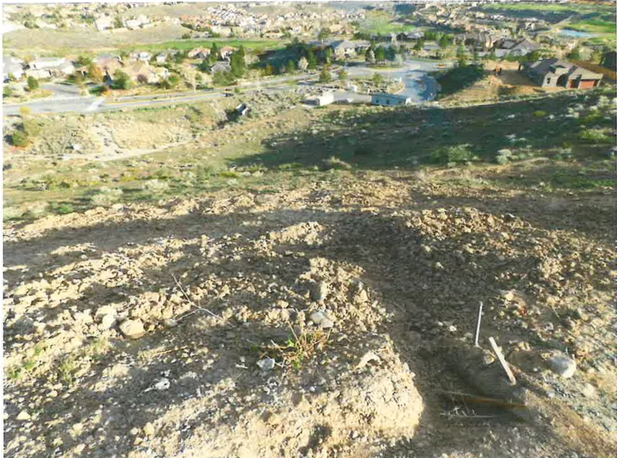
Figure 30 – Hillside Erosion Issue. Installation of Sediment Rolls and Re-Seeding would be the recommended fix; however, given the previous re-seeding issues, installation of rip rap at this location may be the preferred fix. A failed sediment roll can be seen in the bottom right corner.
