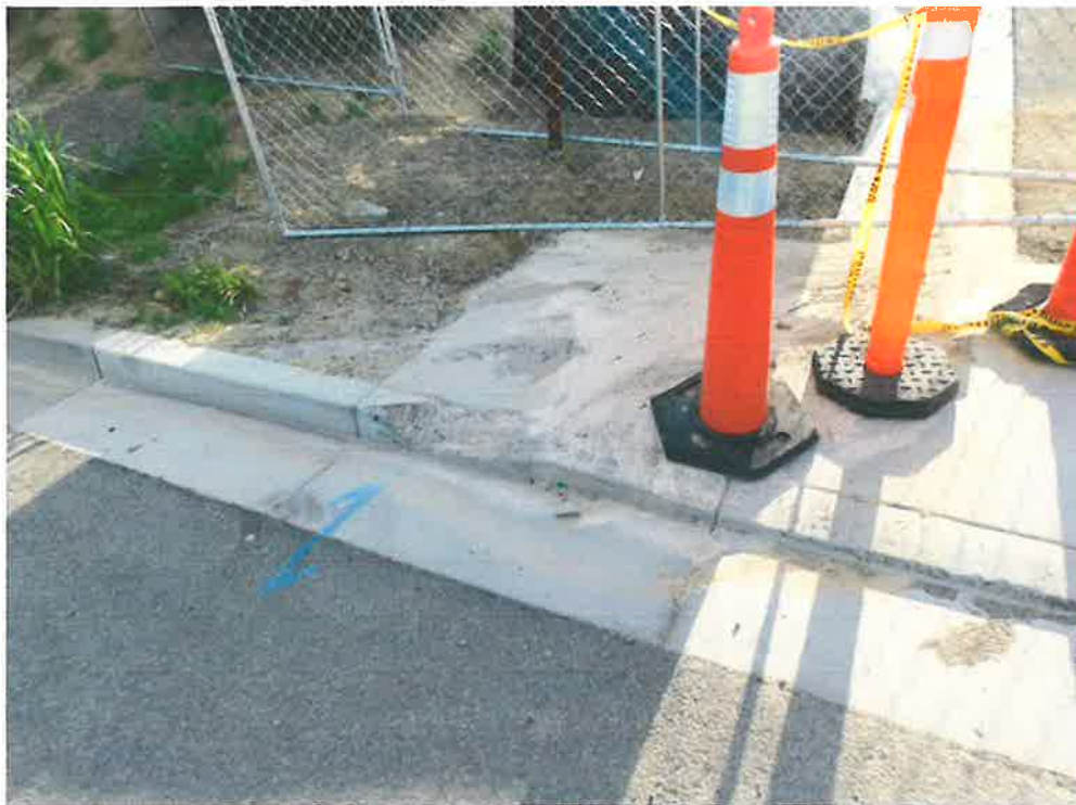
Figure 35 – Damaged Curb for Replacement
