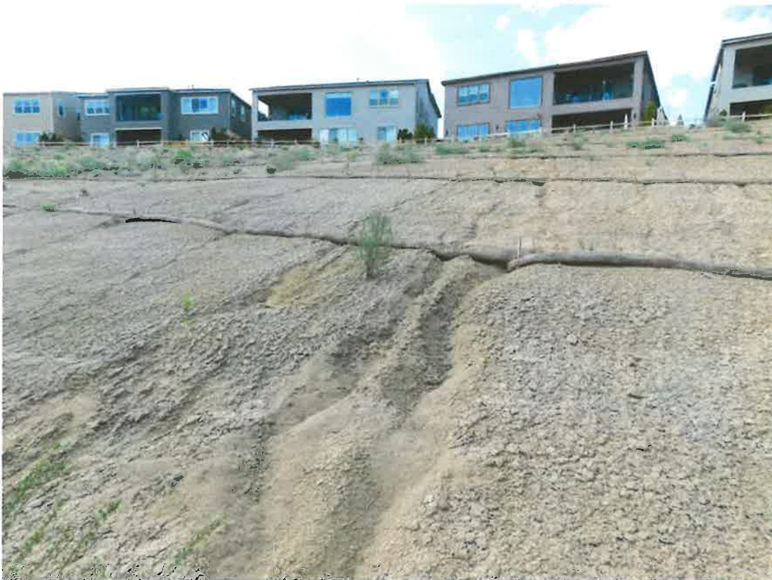
Figure 43 – Erosion Issues are Apparent due to Lack of Proper Revegetation / Re-seeding efforts
