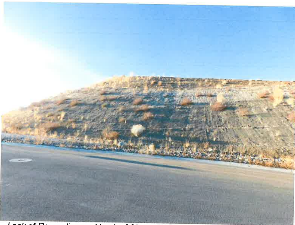
Figure 49 – Lack of Reseeding and Lack of Slope Stabilization Treatments still prevalent in open space North of Graycliff Ln. Photo Taken January 25, 2024.
