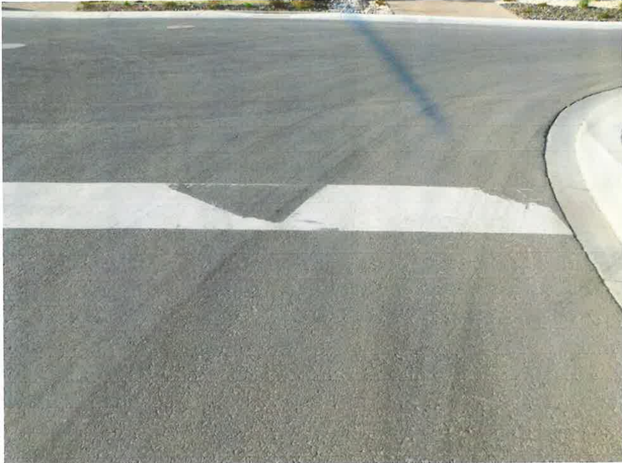
Figure 38 – Stop Bar which needs Re-striping at the corner of Iron Sky Ct and Crossbridge Way
