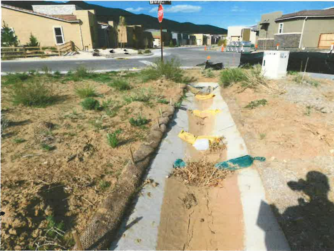
Figure 42 – Large amount of sediment and debris in Valley Gutter.
