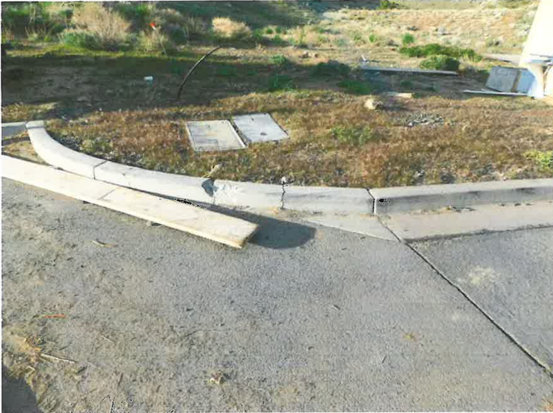
Figure 36 – Another Portion of Damaged Curb Set for Replacement
