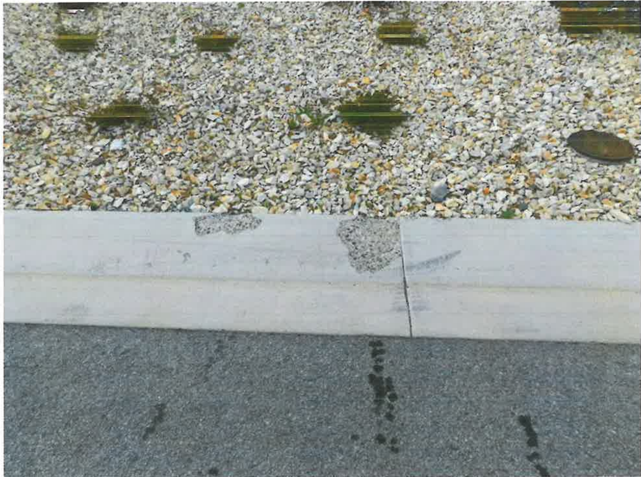
Figure 23 – Damaged portion of Type II Curb should be replaced. Recommend saw-cutting old curb and removing, before replacing with new Type II Curb. Appropriate expansion joint should be placed between old and new curb.
