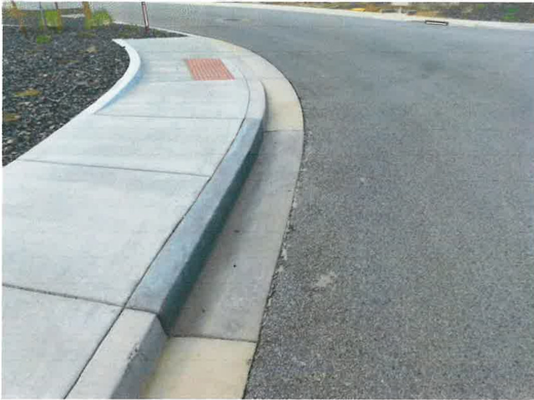
Figure 21 – New Curb and Gutter observed around "The Cliffs" Roundabout
