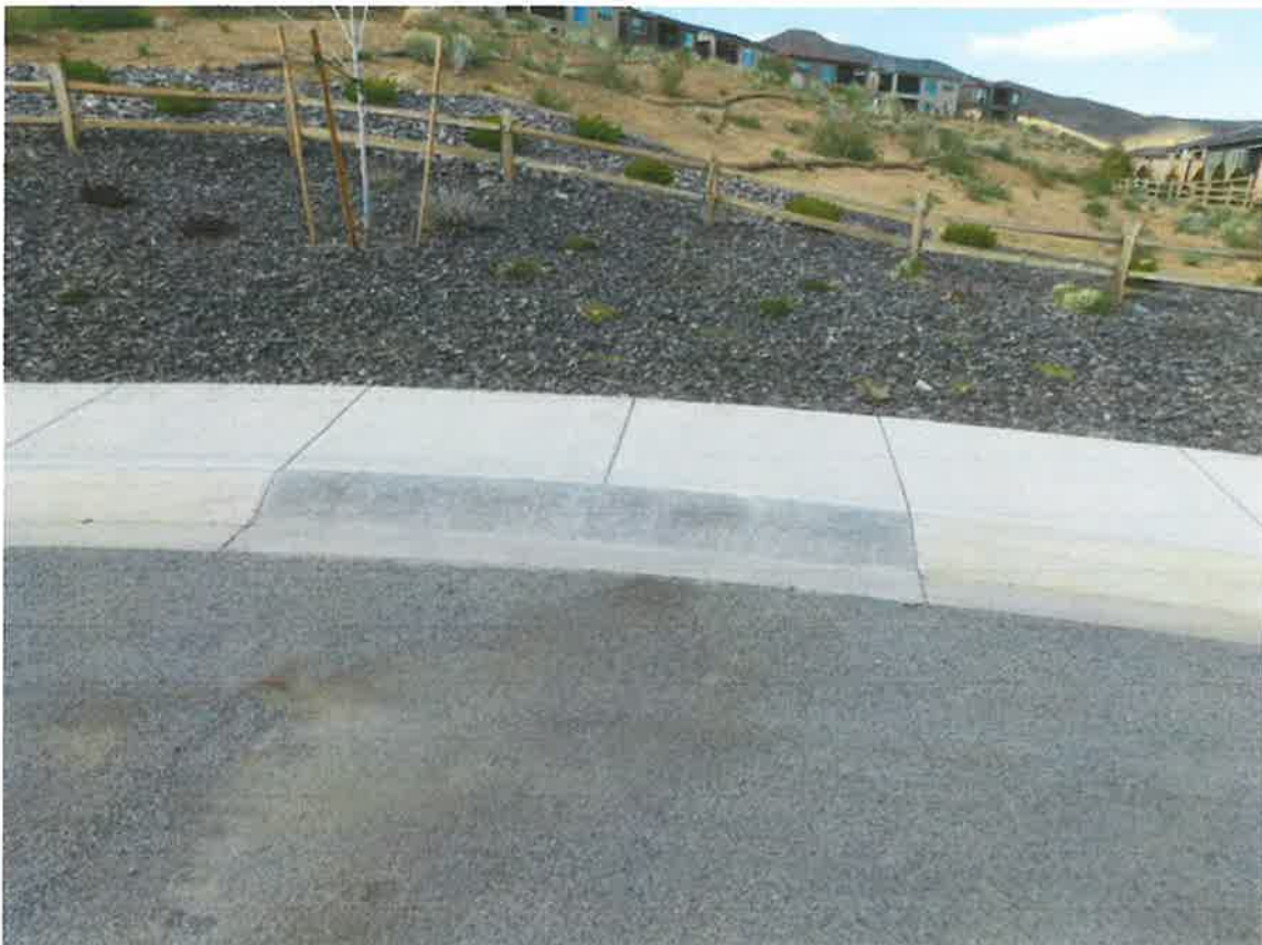
Figure 22 – Another Section of Replaced Type II Curb observed around "The Cliffs" Roundabout
