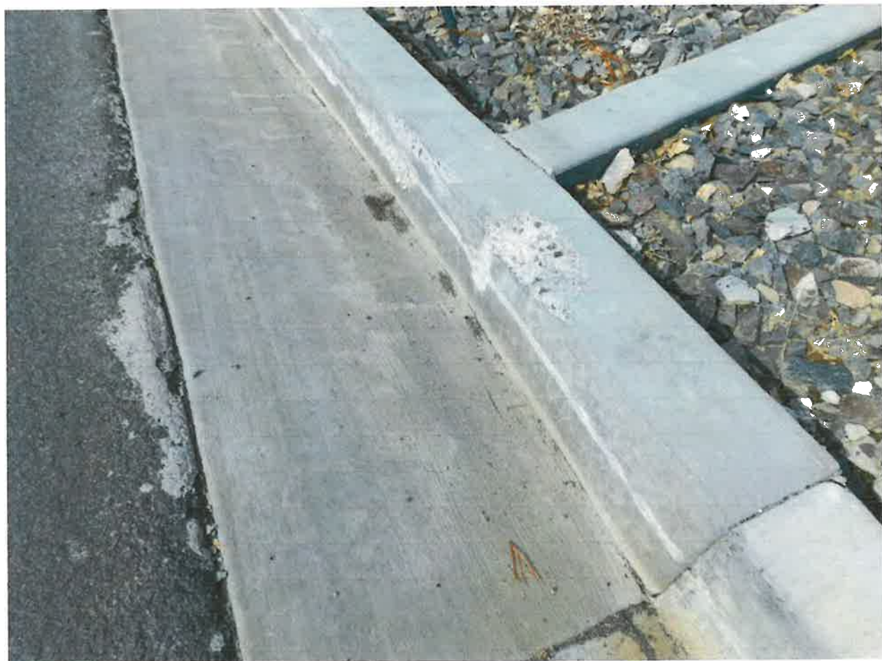
Figure 19 – New Concrete Curb is already damaged. Recommend pulling special inspection records for this batch of concrete. Concrete curb and gutter may need to be replaced.
