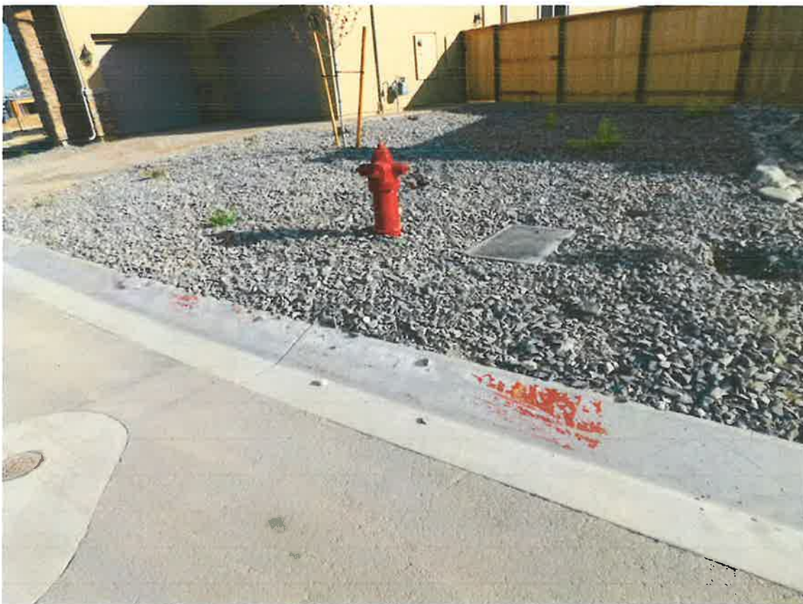
Figure 25 – The worst observed red striping in front of all fire hydrants.
