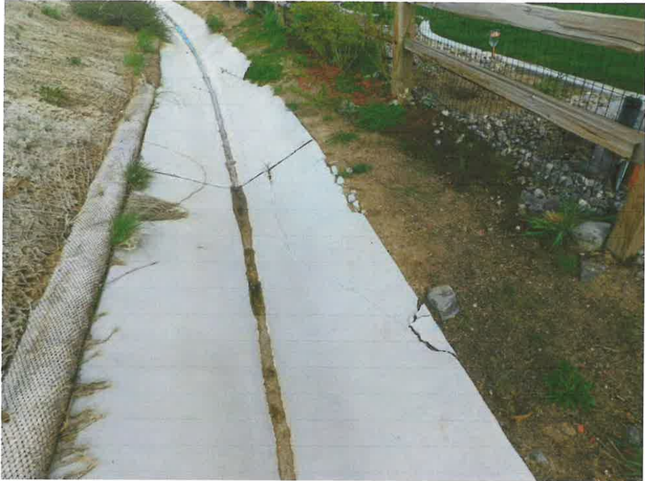
Figure 45 – Valley Gutter is Cracked and Beginning to Fail in open space, north of Graycliff Ln.
