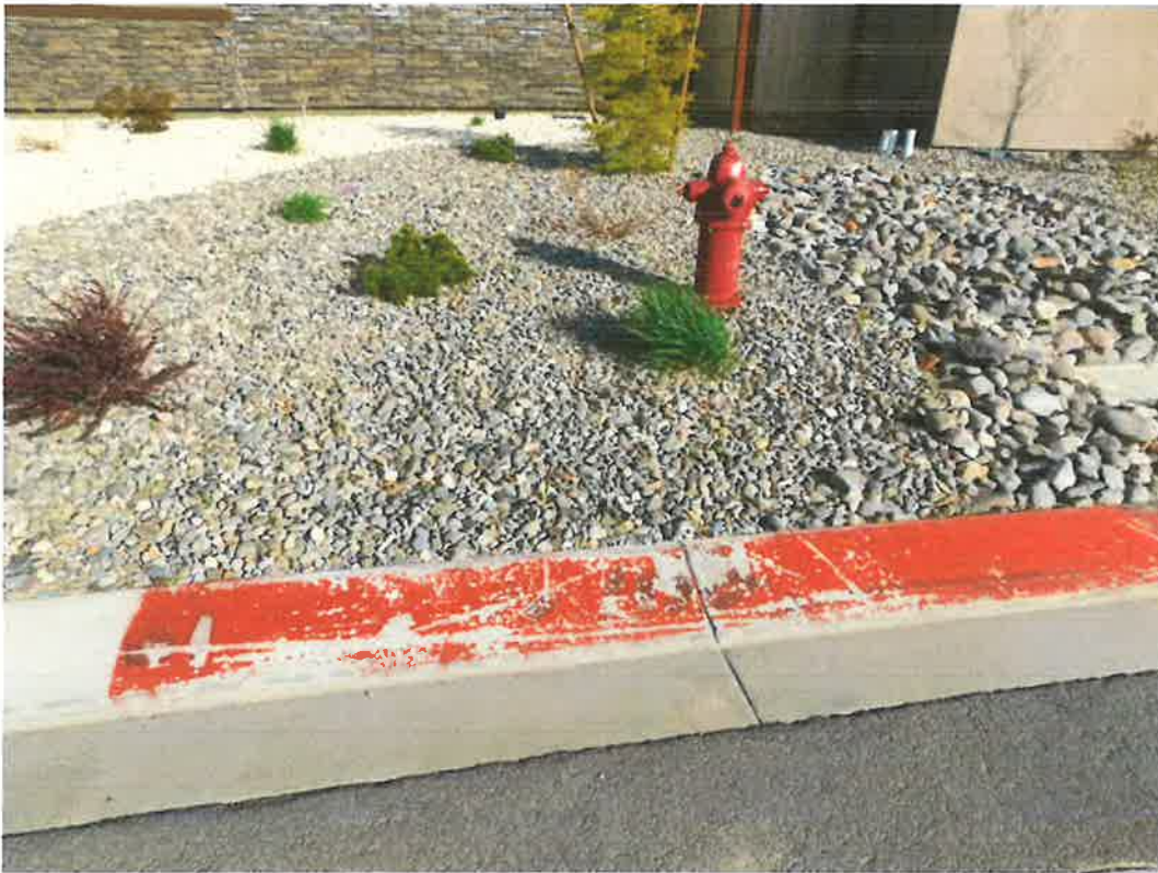
Figure 24 – Typical failing red striping in front of fire hydrants. Recommend all Fire Hydrant Areas are re-striped. Some areas have peeling paint and should be scraped before applying new paint.
