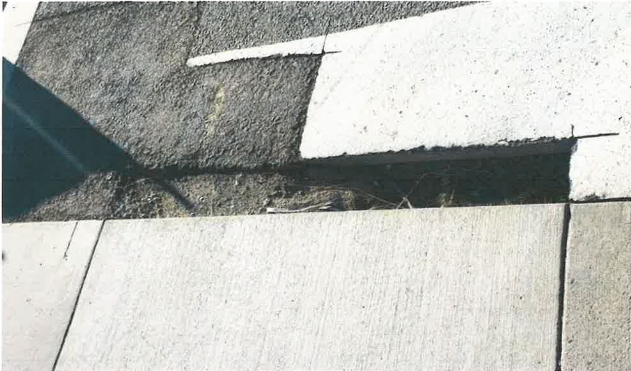
Figure 34 – Here is a zoomed view of the open sawcut area provided to our office. Pursuant to information provided to our office by Nancy Kerry of Somerset, this temporary fix was not performed by Toll Brothers. This area will need to be filled in with cold patch until a proper fix can be performed.
