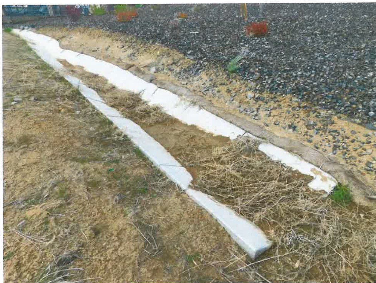
Figure 16 – Erosion Issues have not been fixed at this location and only worsened. The slope should be cut to a less steep grade and all soils above the valley gutter should be covered by rip rap. Additionally, the valley gutter should be cleared of sediment and debris after said repairs.
