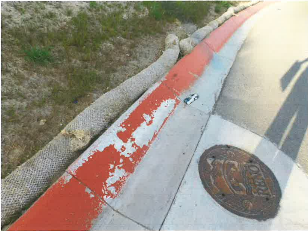
Figure 40 – Curb along the north side of Blue Pinion Dr should be re-striped along its entirety.
