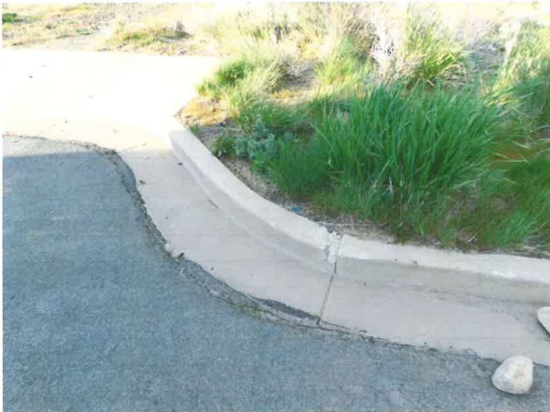
Figure 37 – Another Portion of Damaged Curb which should be fixed.
