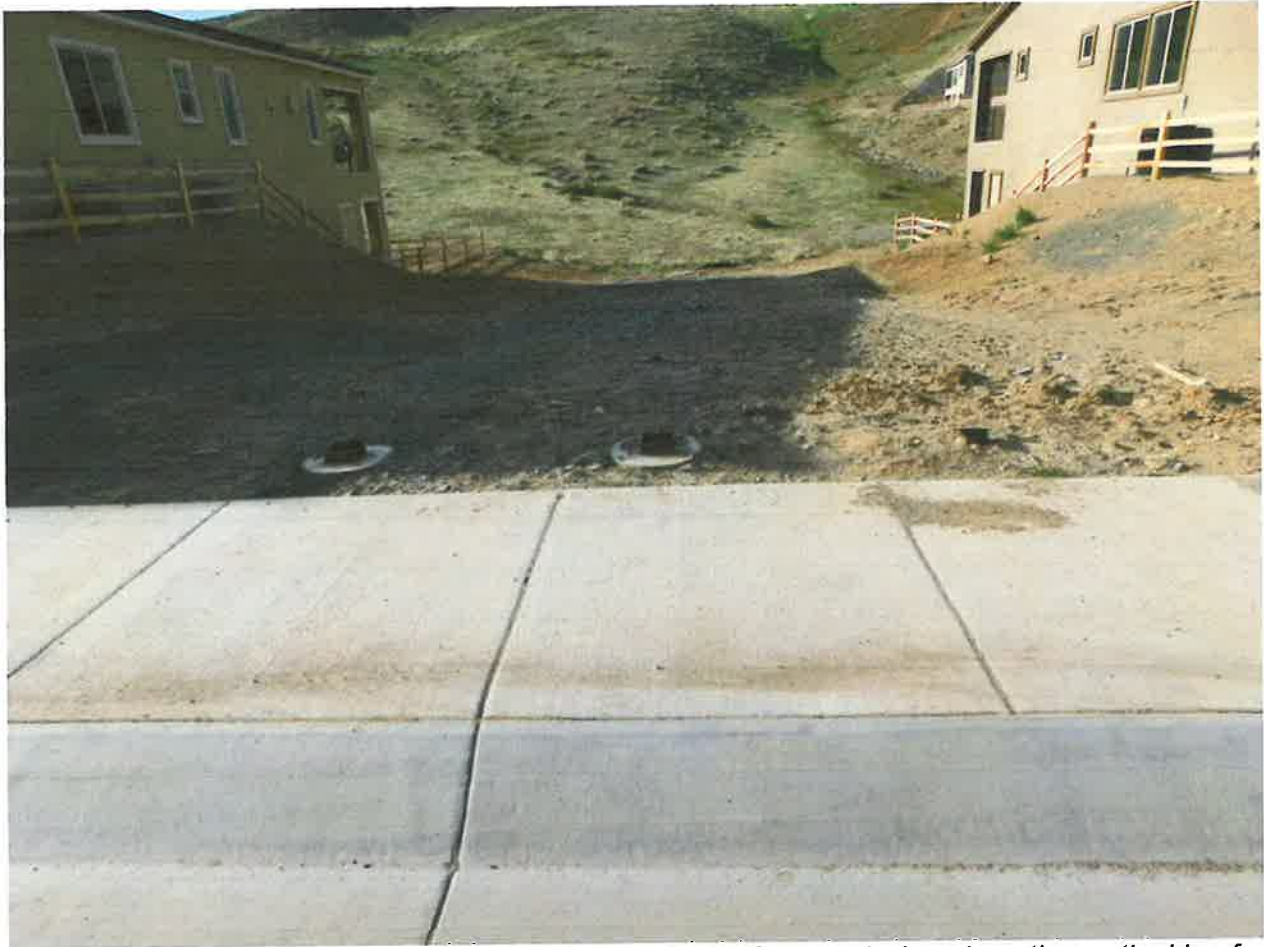
Figure 27 – The traffic barriers to prevent vehicular traffic are missing along the north side of Wild Skies Way are missing and need to be replaced.
