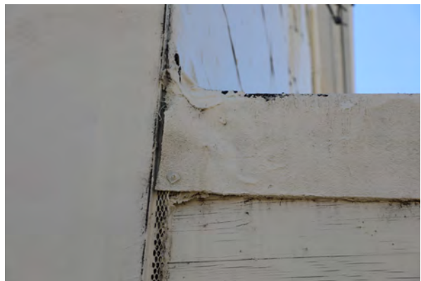
Figure 12: Exposed stucco lath between northwest addition and the temporary wall and roof of the unfinished west addition
