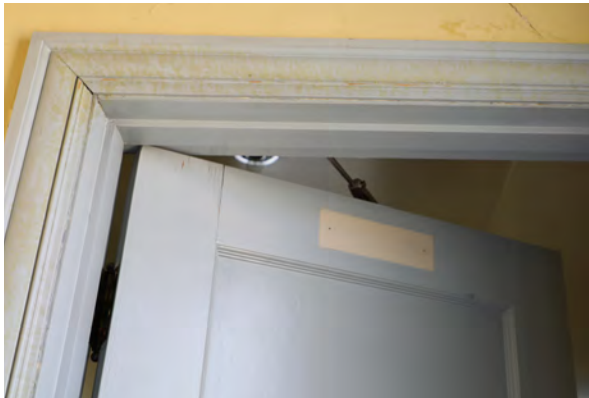
Figure 26: Missing paint at the top rail of the Men's Restroom (Room 105) door and yellow residue visible at the trim
