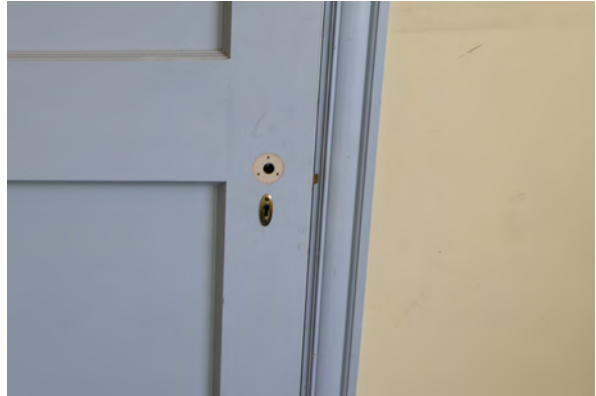
Figure 28: Missing hardware at Door 1-05
