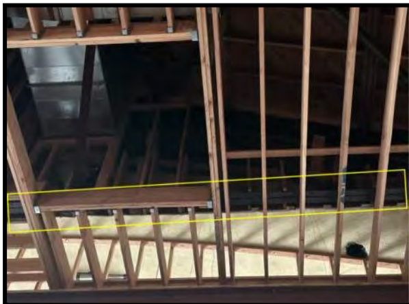
Figure 15 Exposed base of roof truss from Stage.
