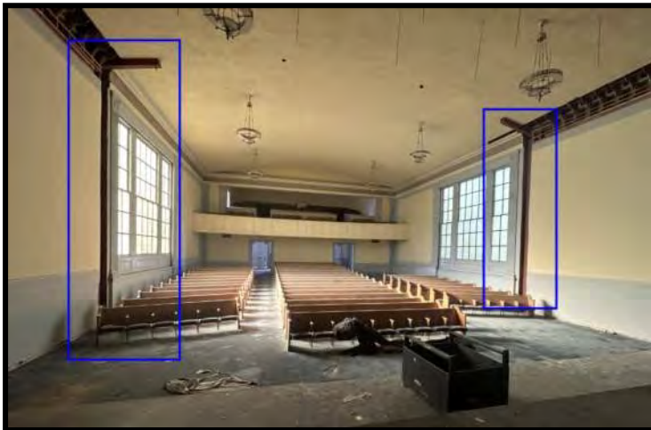
Figure 19 View of the steel TS7x7x1/4 columns from the stage.
