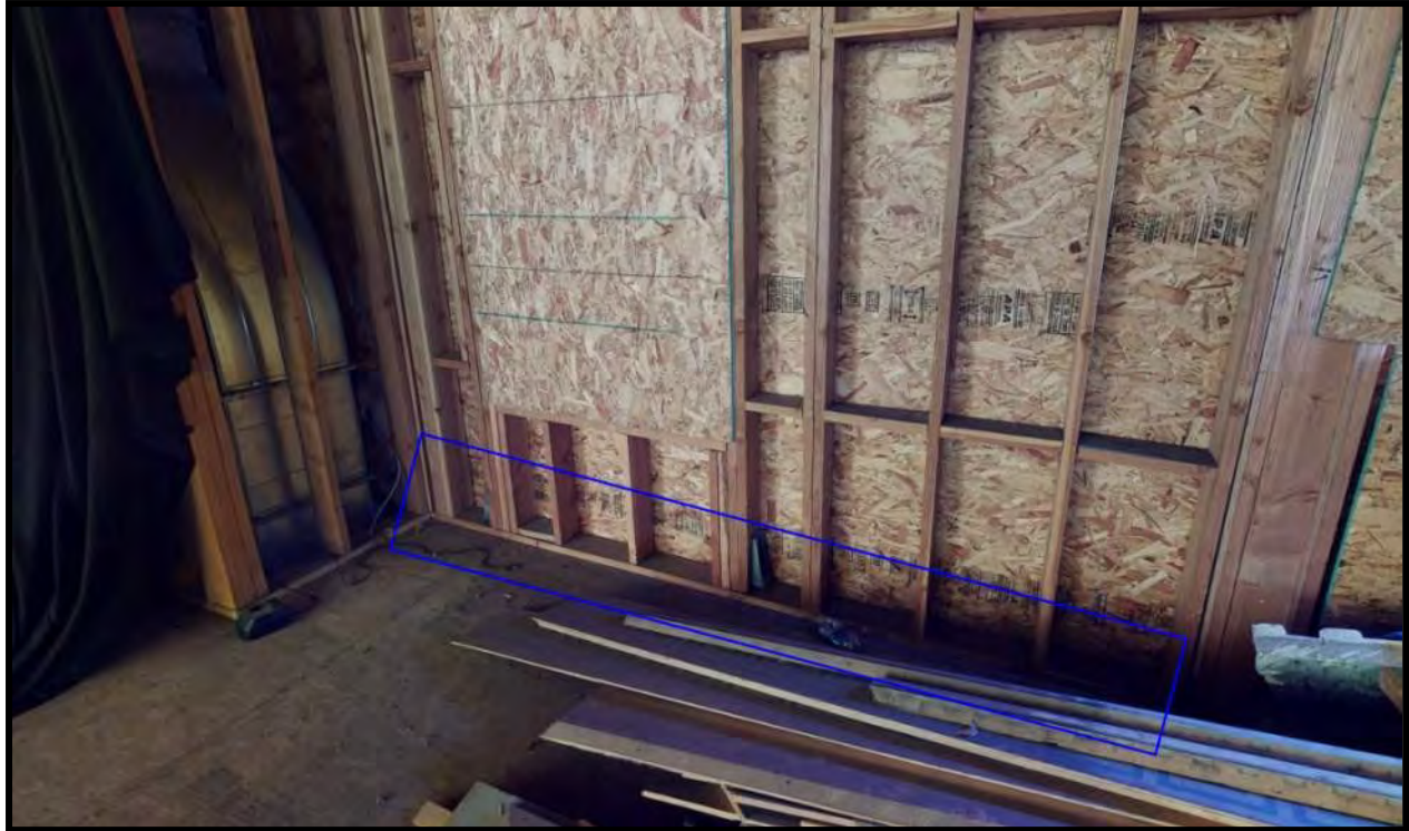
Figure 28 View of missing sill bolts at the north wall of the stage.
