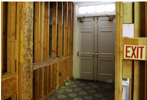
Figure 27: Unfinished construction at the East Entry (Room 109) showing rough opening and wall framing
