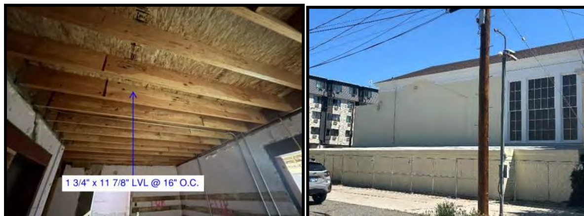
Figure 13 View of the 2002 first floor framing from the basement (left). View of the 2002 sleeper floor from the exterior of the building (right).
