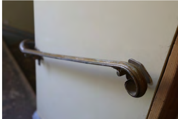
Figure 40: Stair handrails lack ADA compliant extensions, and are not at the proper height
