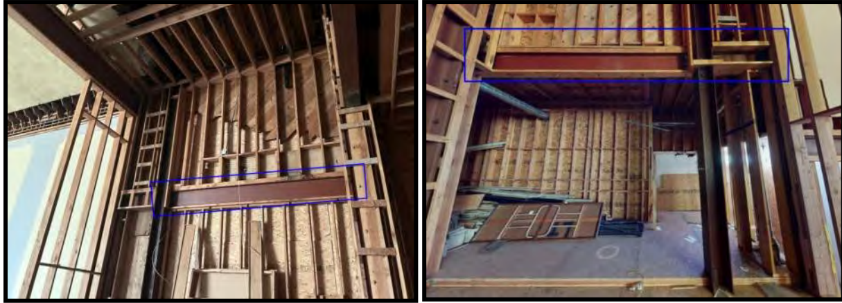
Figure 18 View of west (left) and east (right) steel framing above the stage.
