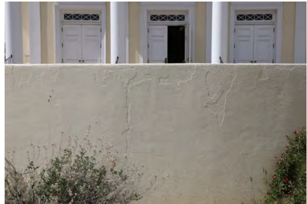
Figure 08: Paint loss telegraphing through new paint coating at south face of the south terrace
