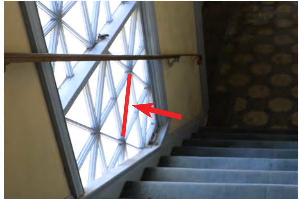
Figure 16: Missing interior muntin at Window 1-12
