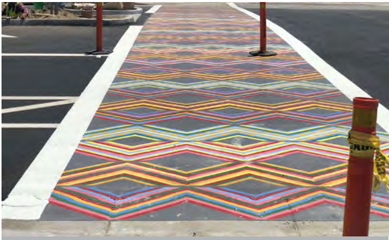
Crosswalks-Ennis Flint Traffic Patterns Thermoplastic Inlay with pattern lasts up to 10 years with normal wear
